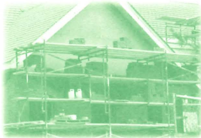
June 2000, Brickwork in Progress
