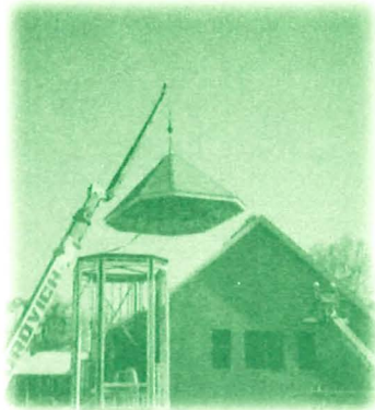
Spring 2000 Placement of Tower Roof
